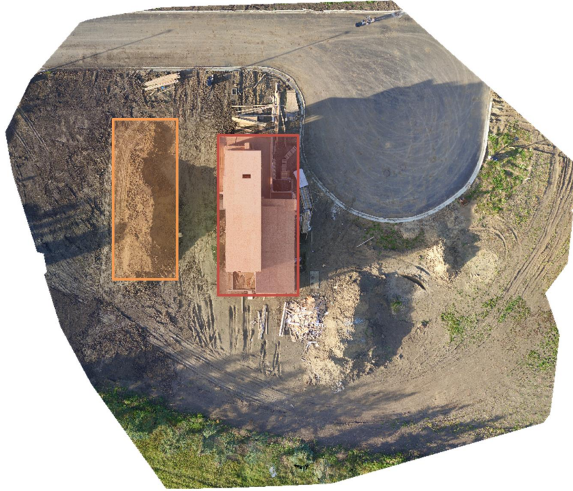
Figure 4.9: Example of reserved areas. The area for stockpile and the building cannot serve as hauling road after grading.
