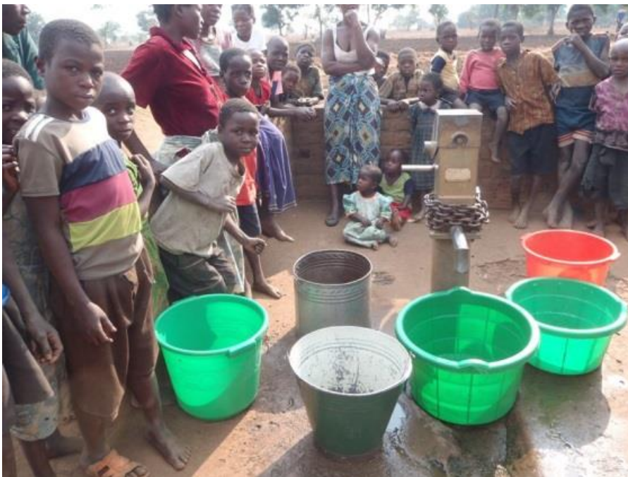
A hand pump managed by a local mission school. The chains serve to lock it at night to prevent vandalism and theft (Dedza area)
