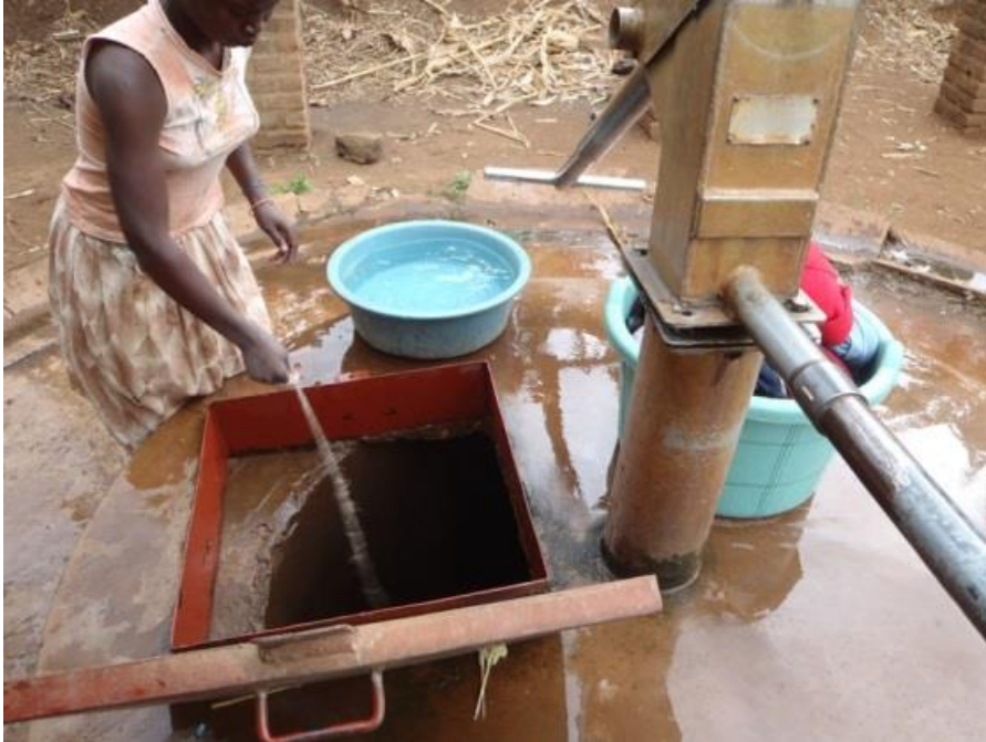
Here a woman demonstrates how a protected well can be accessed with a rope and bucket if the hand pump is inoperable. This is better than an open well but in many cases this becomes the default condition in the village (The temporary wire binding in Kalonga Village was insufficient and did not last while bolts were being sourced)
