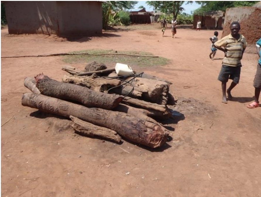
A crudely covered open well in a village; a serious health and safety threat (Filimoni area)
