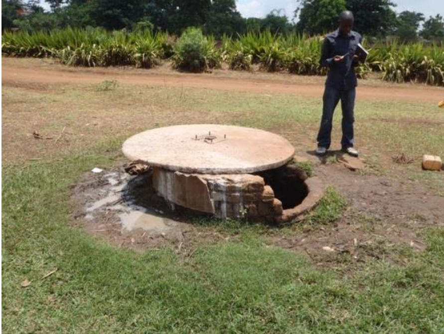
A covered well that lacks a pump and has been modified to for rope-and-bucket use (south of Mitundu).
