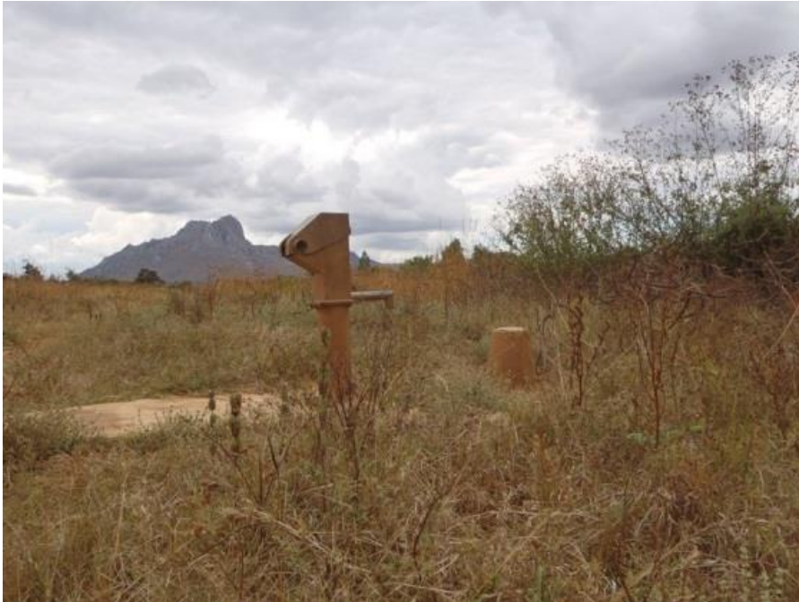
A common sight in Malawi – dysfunctional and stripped hand pump (near Nkhoma)
