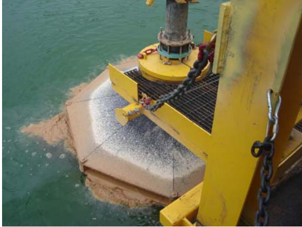
Figure 10. Full scale, octagonal tremie/diffuser being deployed at McClean Lake.
