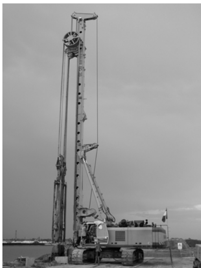
Figure 7. CSM Machine mounted on BG2
