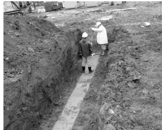
Figure 3. Top of excavated CSM wall
