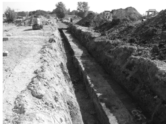
Figure 15. Excavated top of Cut-off Wall
