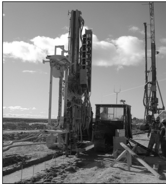
Figure 19 UBW 09 drilling jet-grouting Holes
