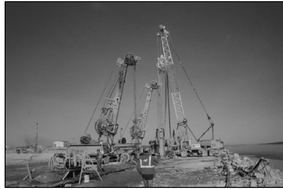
Figure 19. Cutter and Grab used in Panel Wall Construction
