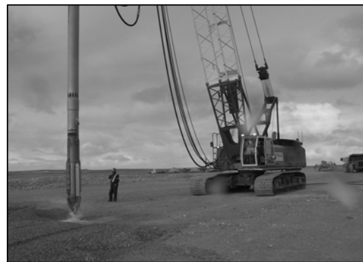
Figure 17. Compaction with TR75 deep Vibrators
