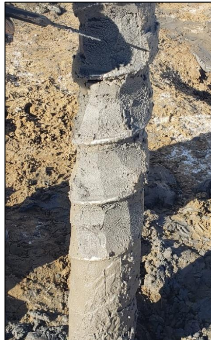
Figure 3-4: Auger Stem
