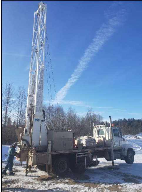
Figure 3-1: Typical Boring Rig with Solid Stem Auger
