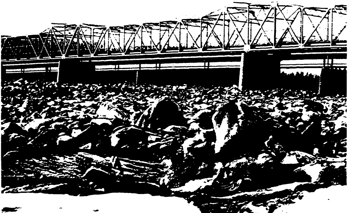
Figure 1-3. Ice jam at MacEwan Bridge in 1977.
