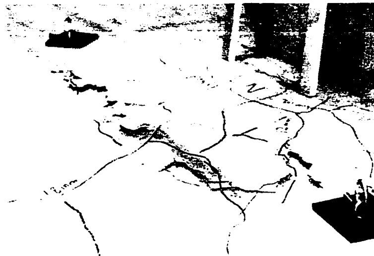
Figure B.14 Cracks at Failure – Control Specimen (Looking South-East)
