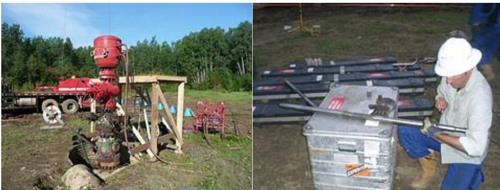
**(Upper left)** Rig setup and the removal of tubings from the borehole prior to logging.
