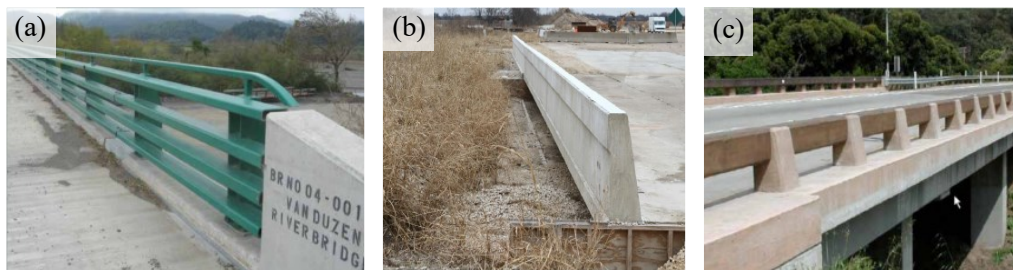
Figure 2.1 Types of bridge barriers. (a) Steel barriers (Caltrans), (b) Continuous concrete barrier (Sheikh et al. 2011), and (c) Concrete barrier with openings (Caltrans).
