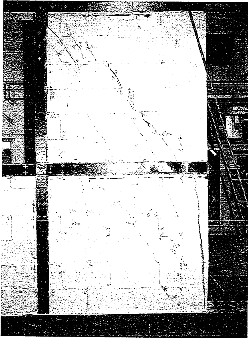
Photo 4-3 Crack Patterns for Wall 3
