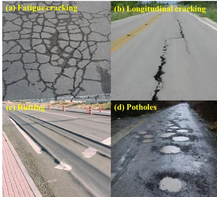
**Figure 2-2.** Distresses in flexible pavement [28]
