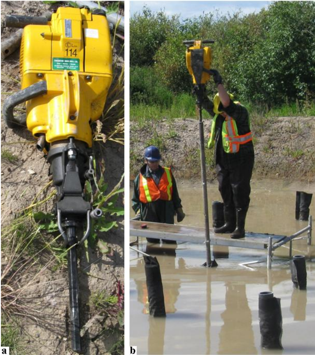
Figure 3-5: a: Gasoline powered Pionjar 120 portable drill used for coring; b: Driving aluminium tube into the clay till at the bottom of the Infiltration Pond using gas powered drill.
