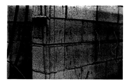
Plate 5.15 Crack at Interface of Beam EB2 and Supporting Wall
