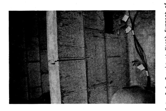
Plate 5.6 Cracks at North Support of Beam RB1
