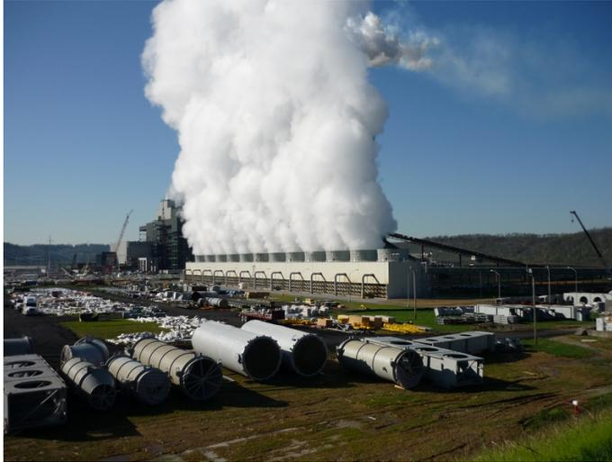
Figure 1.8: Visible plumes above a single row of cooling tower cells. (Photo used with permission of International Cooling Tower Inc.)
