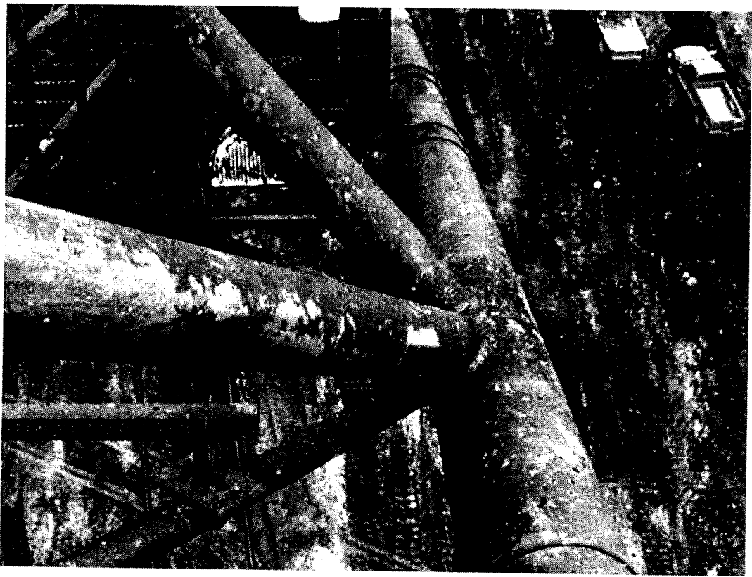
Figure 6.2 Cluster in dragline boom, the transition in question is 250 mm away. Courtesy Syncrude Canada Ltd.
