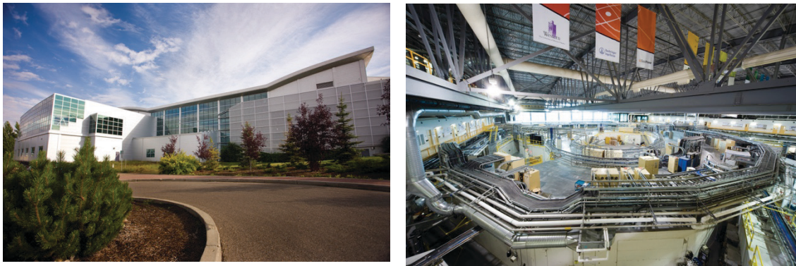
Figure 2.14 The exterior and interior of the Canadian Light Source. (Images courtesy of the Canadian Light Source, Inc.)
