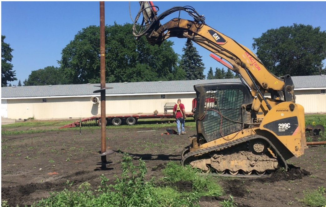
Figure 1-3: Installation of a Double-helix Pile
