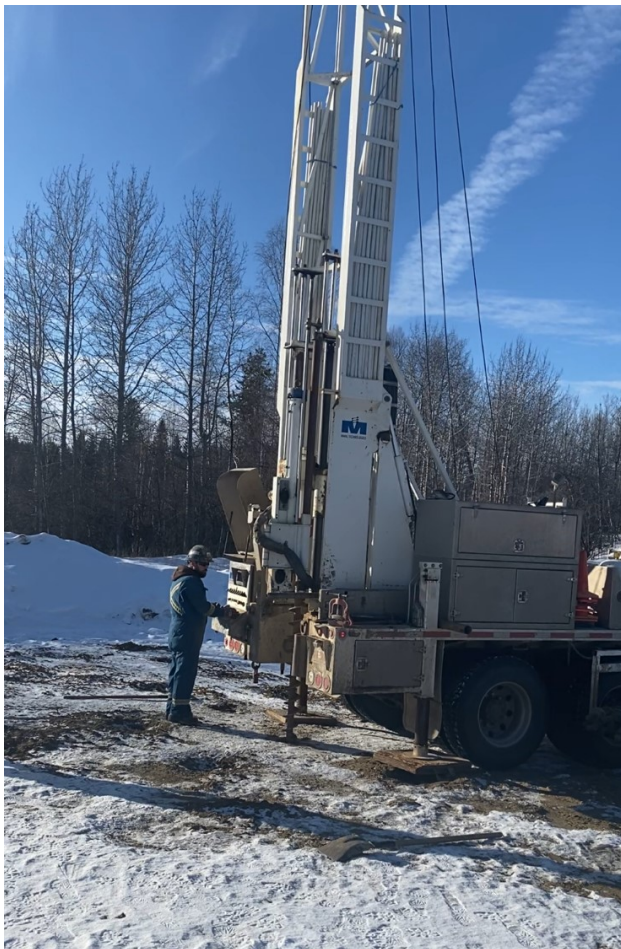
Figure 2-3: Photo of SPT Operation
