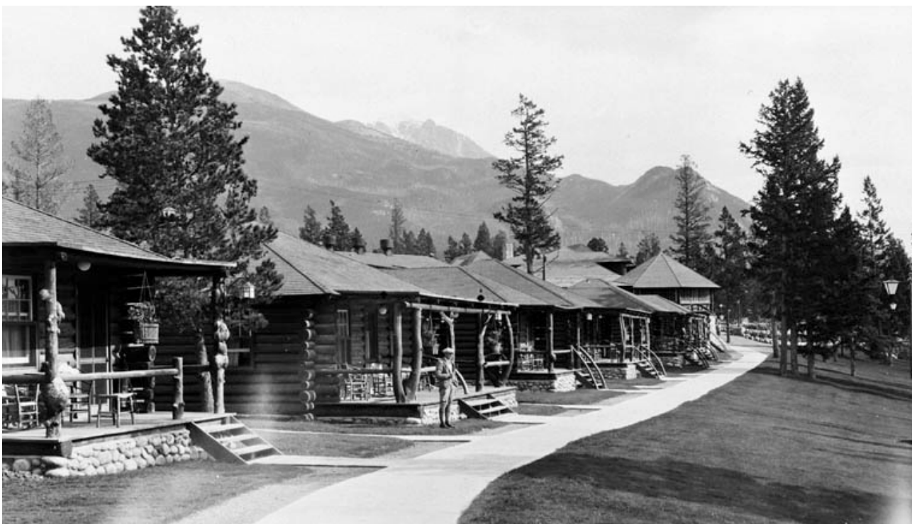
Fig. 24 Sidney Ells, Walkways at Jasper Park Lodge Surfaced with Bituminous Sand, Jasper, Alberta.
