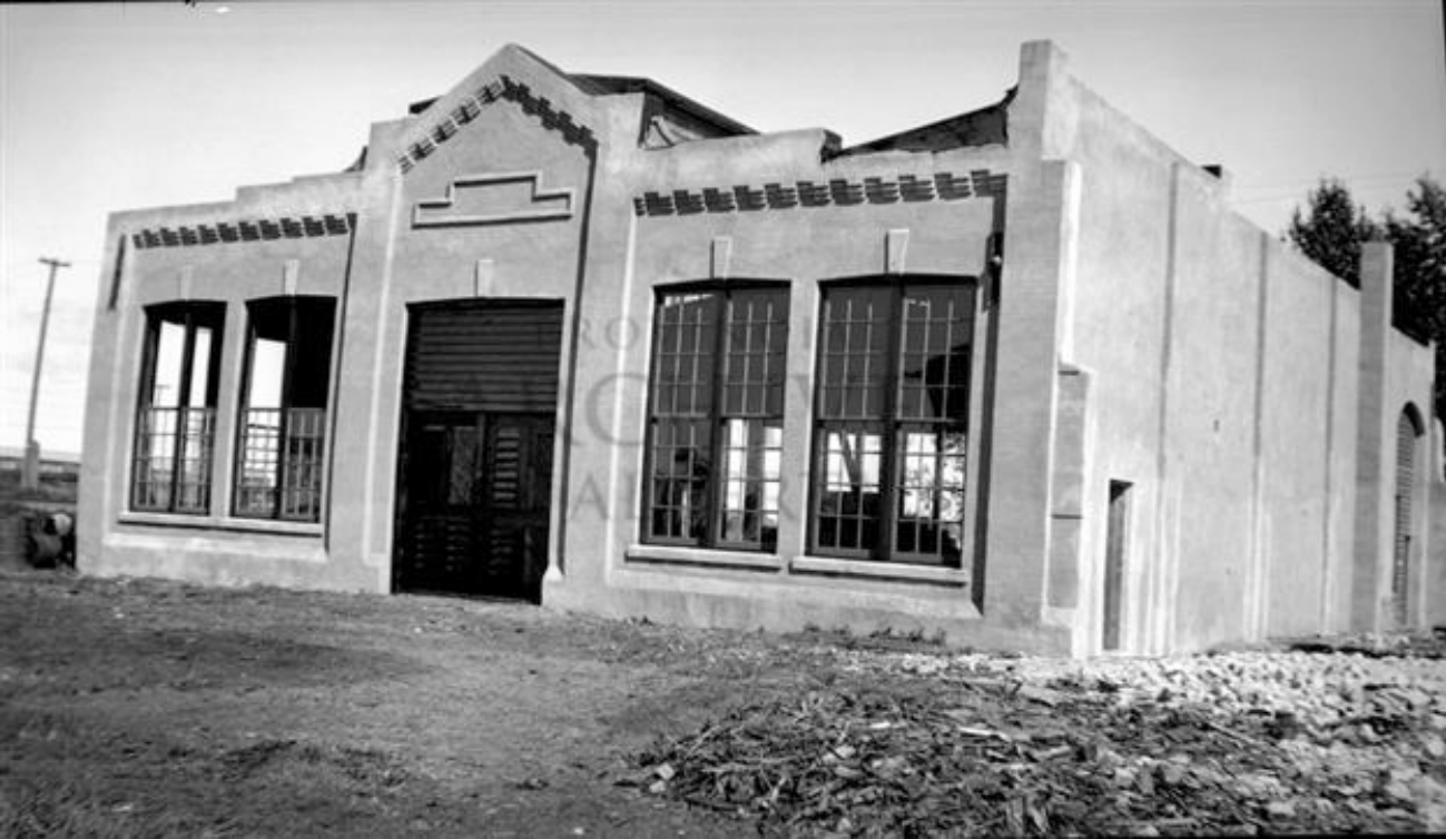
Fig. 27 Robert C. Fitzsimmons, Tar Sands Building Edmonton; View of Exterior of Building Located at 5338-126 Avenue in Edmonton, Alberta.
