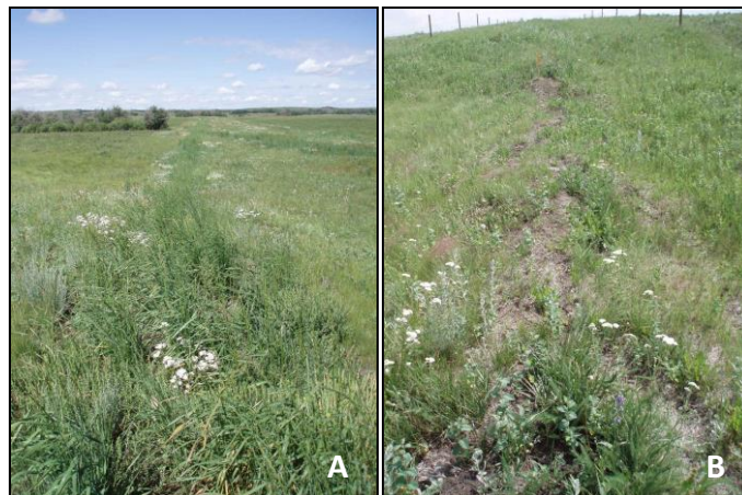
Fig. 1. (A) Plow-in pipeline with topsoil removed, replaced and seeded. Dominated by wheatgrasses. (B) Plow-in pipeline using a bucket plough, left to natural recovery. First year after installation, a south slope with rough fescue, rose, snowberry and other native grasses and forbs.
