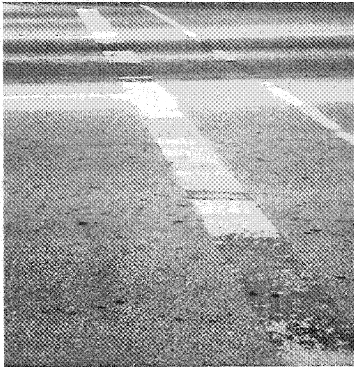
Figure 3.9: Abrasive Wear of Transverse Lines at Low AAWT rates
