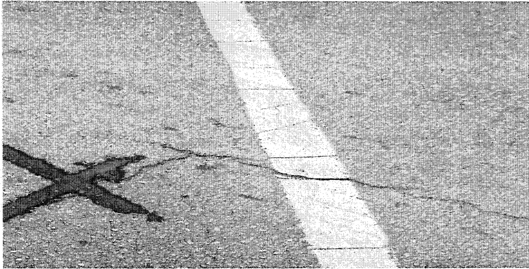
Figure 1.5: Transverse Cracking of Thermoplastic Roadway Marking
