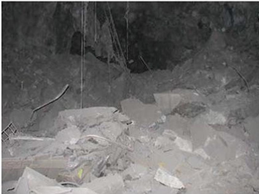
Figure 2.2. Displaced materials at the Copper Cliff mine's 3880 level after an earthquake on 25 March 2008, which shotcrete ground support failed to contain (Morissette et al., 2017), CC BY 4.0
