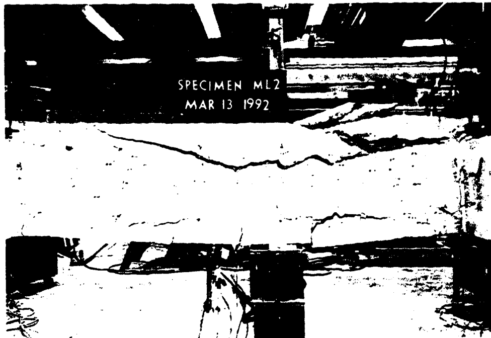
Figure 4.17 Typical Medium Lower Concrete Strength Beam After Failure
