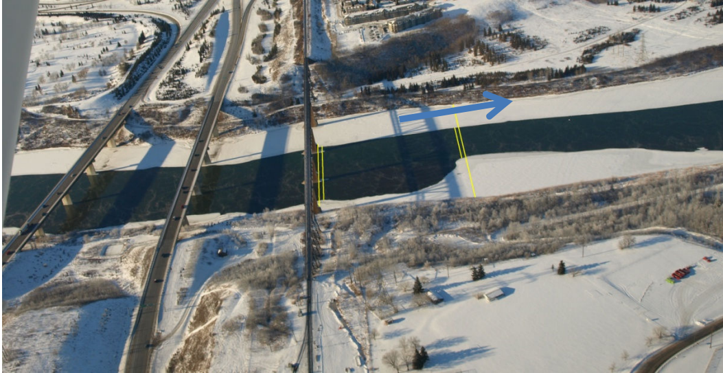
Figure 4-13. Aerial photograph taken 24-Jan-08 illustrating constriction downstream of Highway 16 Railway bridge.
