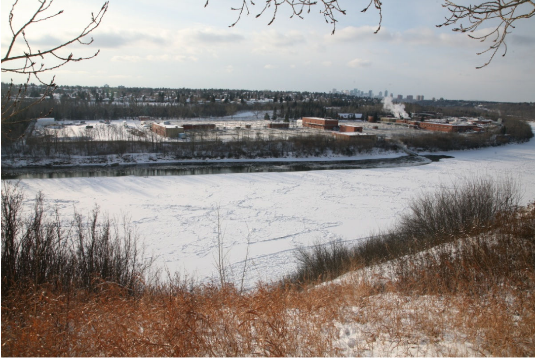
Figure 2-2. Picture of GBWTP outfall and the upstream head of the open lead it creates.
