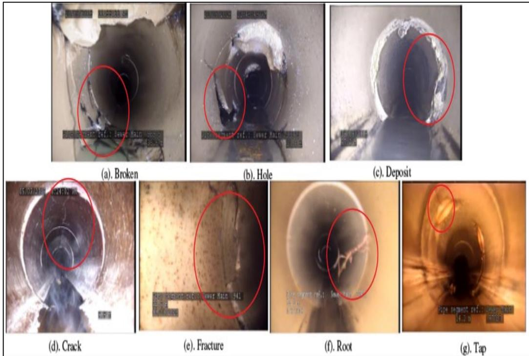
Figure 2. 13: Examples of defects and example of a tap in sewer pipes (Yin et al. 2020)
