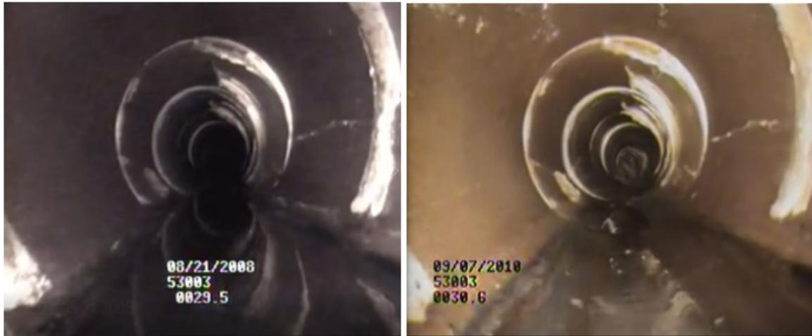
Figure 3. 2 Time-series sewer pipe defect image in 2008 and in 2010
