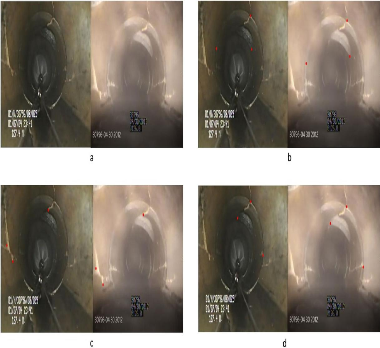
Figure 3. 6: a) A pair of matching images from pipe segment 30796, b) The first pair of matching areas, c) The Second pair of matching areas, d) The third pair of matching areas
