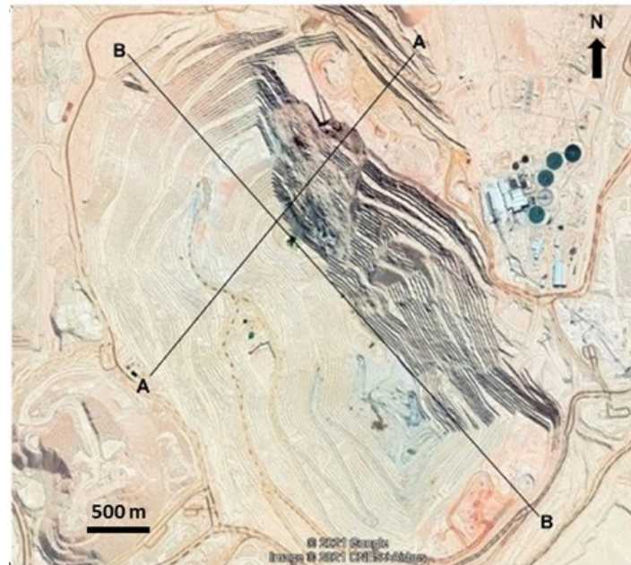
Figure 3-1. Plan view of the open pit case study (modified from Google Earth, 2019). The failure appears as the disturbed area in the northeast corner of the pit, with the longitudinal section line A-A passing through the slide and the transversal section line B-B crossing the toe of the failed zone. The corresponding profiles are provided in Figure 3-2.
