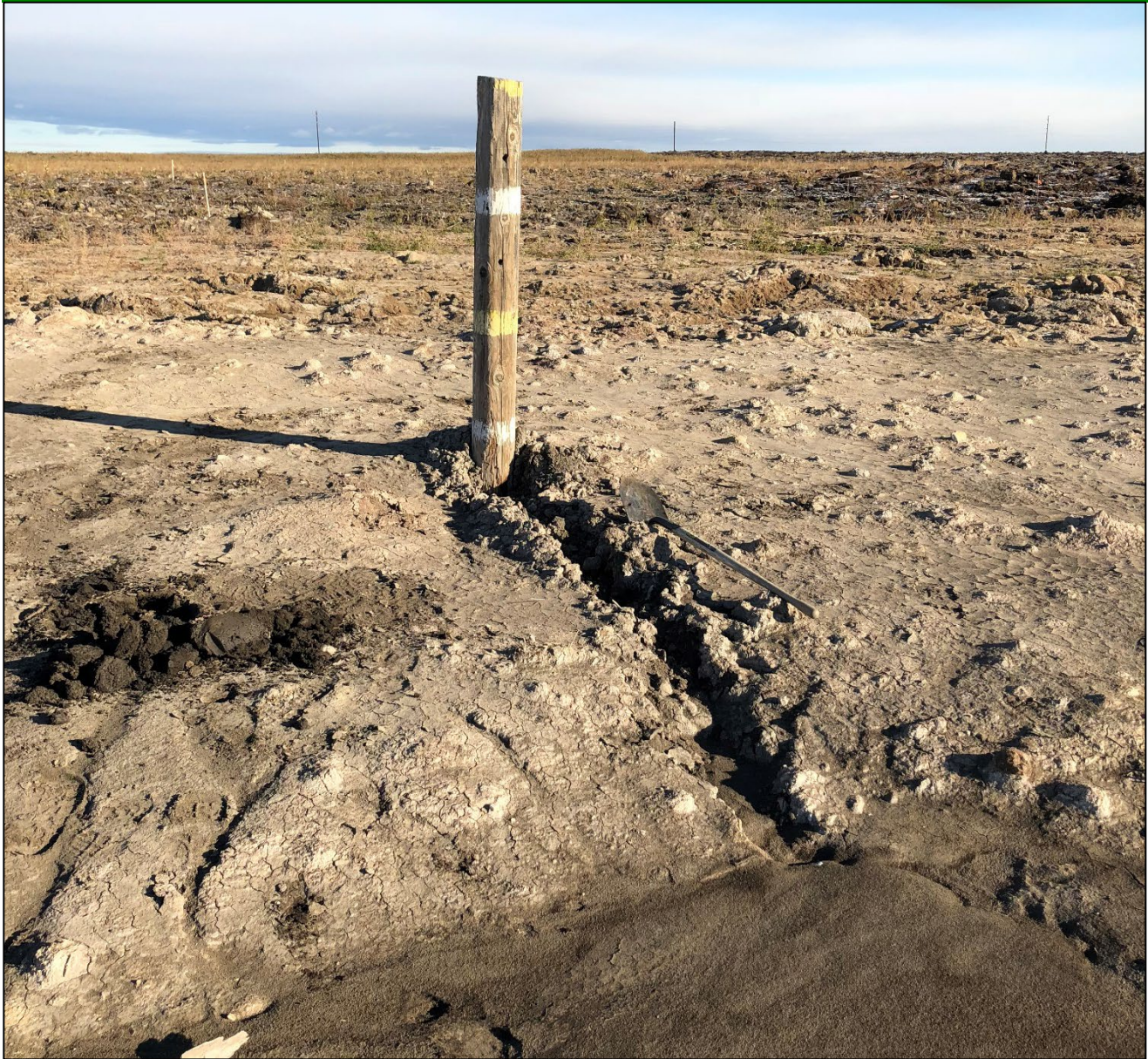
Photo 2. Post installed into overburden beneath cake deposit at margin of reclamation area showing movement of cake deposit away and downslope (south) from reclamation area. Cake is also elevated (forced-up) relative to cake deposit to the south.
