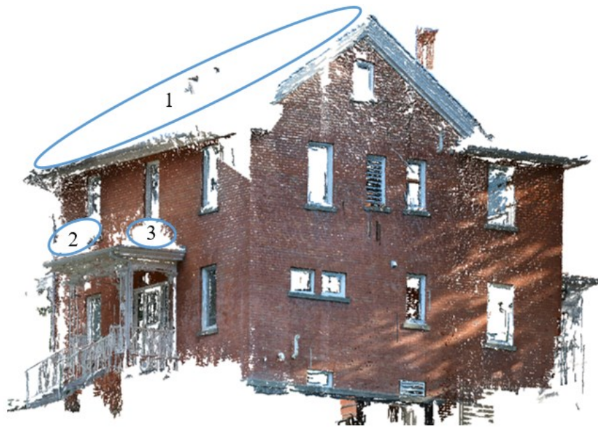
Figure 4-4: Point cloud of the house.
