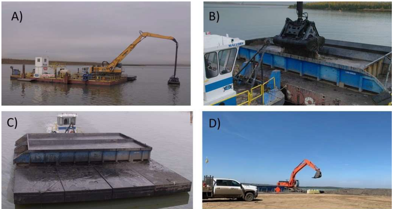
Figure 4-6: 2021 Clamshell dredge operation method A) material handler on dredge collects bitumen and FFT and water from mudline of BML, B) material handler deposits contents of clamshell into hopper barges until full, C) hopper barges are pushed to shore using tugboats, and D) on-shore excavator moves material from hopper barge into wiggle wagons for disposal
