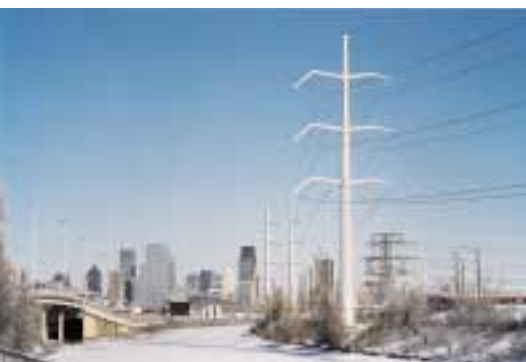
315-kV line on tubular steel poles
