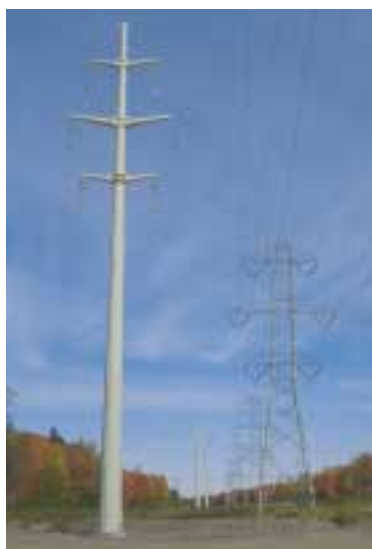
230-kV line on tubular steel poles between Laurentides, Québec and La Suète substations
