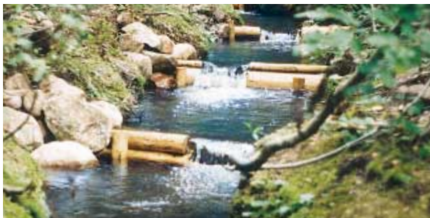
A sample mitigative measure: A fish-pass
