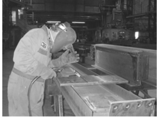
(b) Semi-automatic welding
