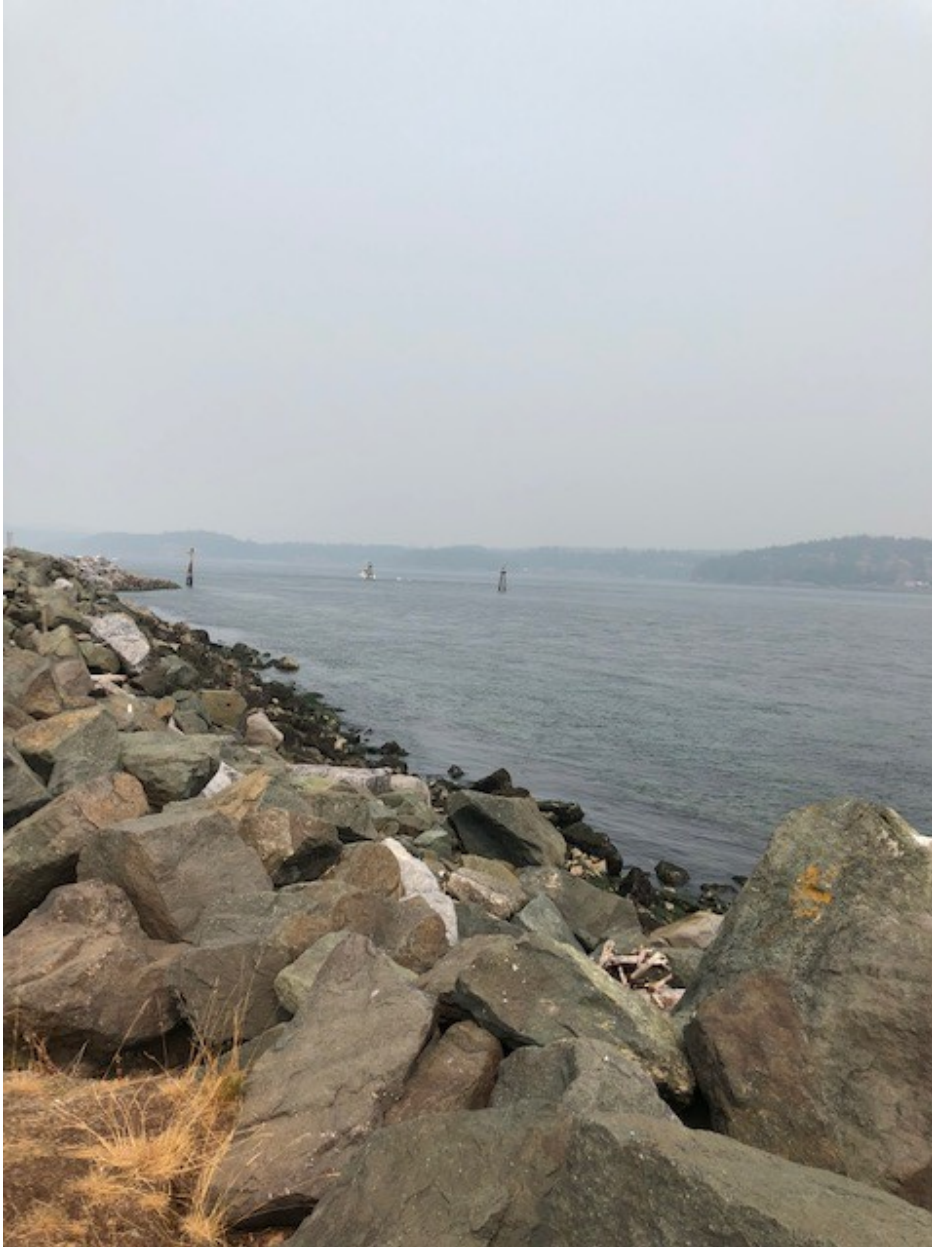
Figure 6- Shoreline armoring in Strathcona Regional District. View of piled rock along the coastline, which serves as shoreline armoring to protect against storm surge and sea level rise. Photo was taken by researcher on August 13, 2018.
