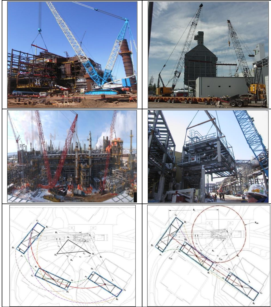
Figure 1.1 Sample Heavy Lifts and Path Planning
