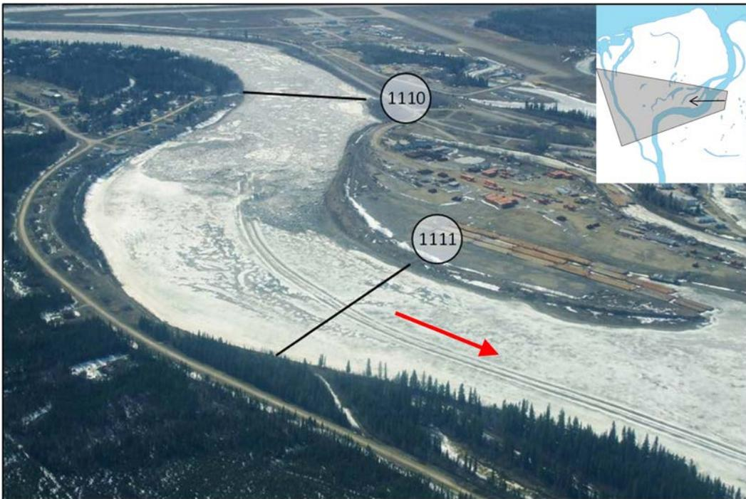
Figure 2.15 Image of ice jam in the East Channel on 3-May-09.
