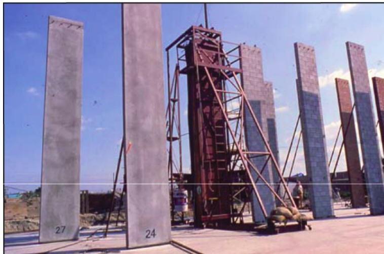
Figure 2.3 – Experimental setup and specimens ready to be tested (1982)
