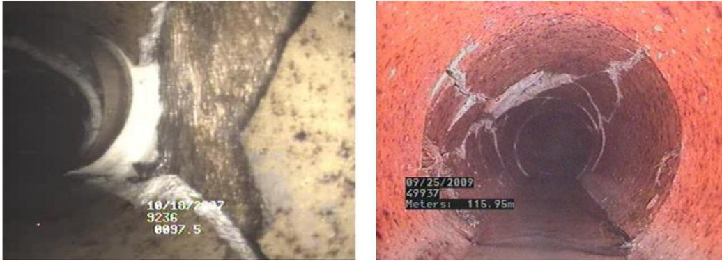
Figure 3.1.No Void Broken Pipe (COE, 2010)
