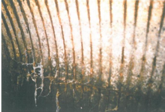
Figure 2.19. Reinforcement Corroded (SRC) (PACP 2001)
