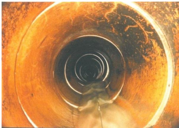
Figure 2.16. Crack – Multiple (CM) (PACP, 2001)
