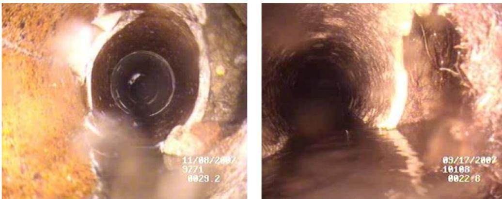
Figure 2.20. Severe Void Broken Pipe (COE, 2010)
