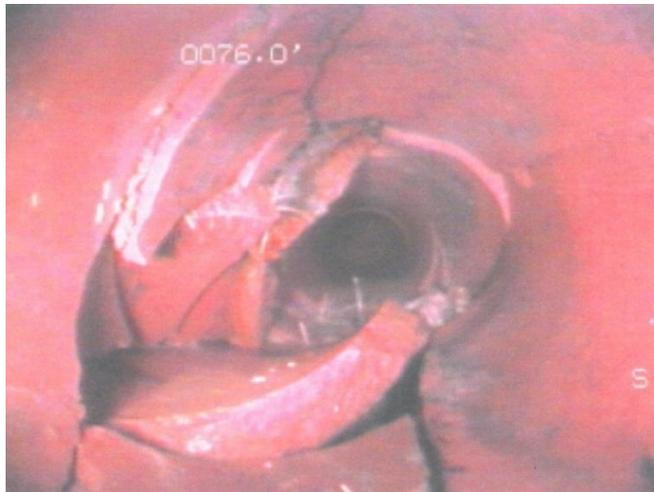
Figure 2.18. Collapsed Pipe (XP) (PACP, 2001)
