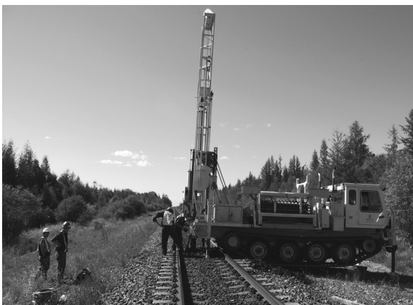
FIG. 6—Surface conditions at Mile 102.0 during installation of instrumentation.
