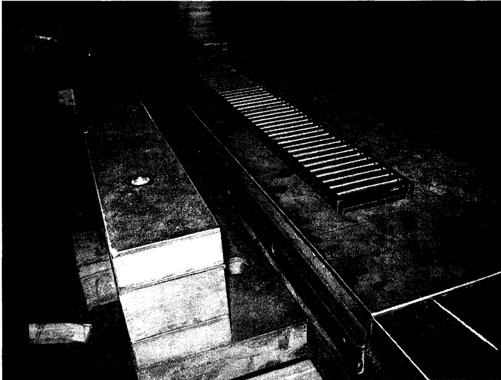
Figure 3.20: Roller Strip – Outer Bearing Plates Removed
