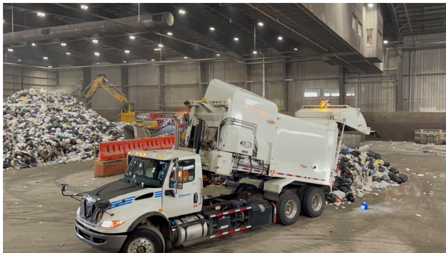
Figure 2: Truck Dropping MSW at Tipping Floor
