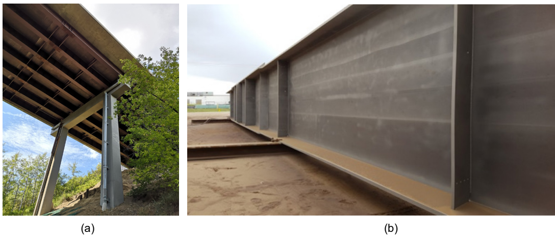
Figure 2.9. Photos of a typical (a) steel girder bridge, and (b) bridge girder ready to ship off to the field from the fabrication shop.
