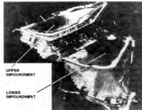
Figure 12. Stava Tailings Dams Before Failure (note impounded water distributions)
