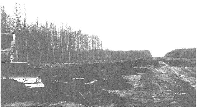
Photo 5. Topsoil replacement on 15 cm treatment.
