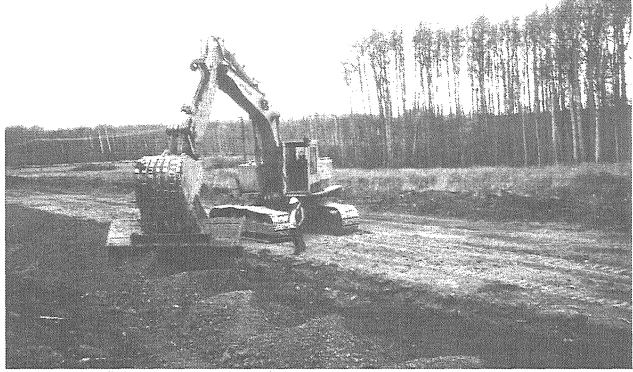
Photo 4. Backfilling the trench with a "flyswatter".
