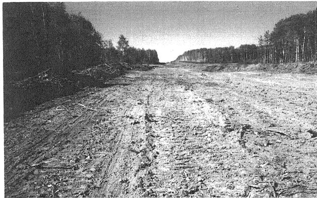
Photo 2. Clearing and stripping completed on 15 cm treatment.
