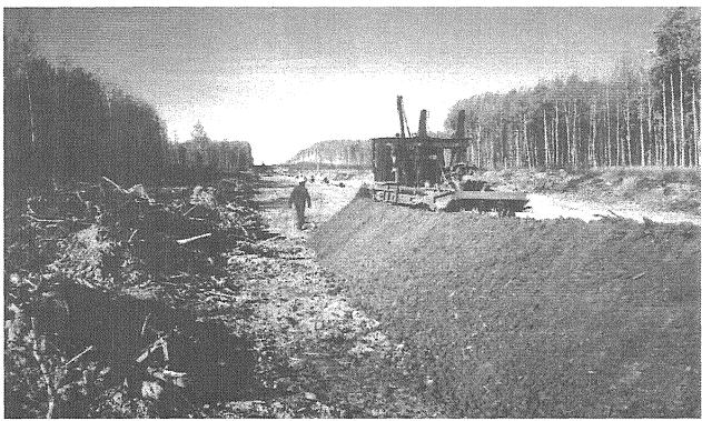
Photo 3. Wheel ditcher at work excavating trench.
