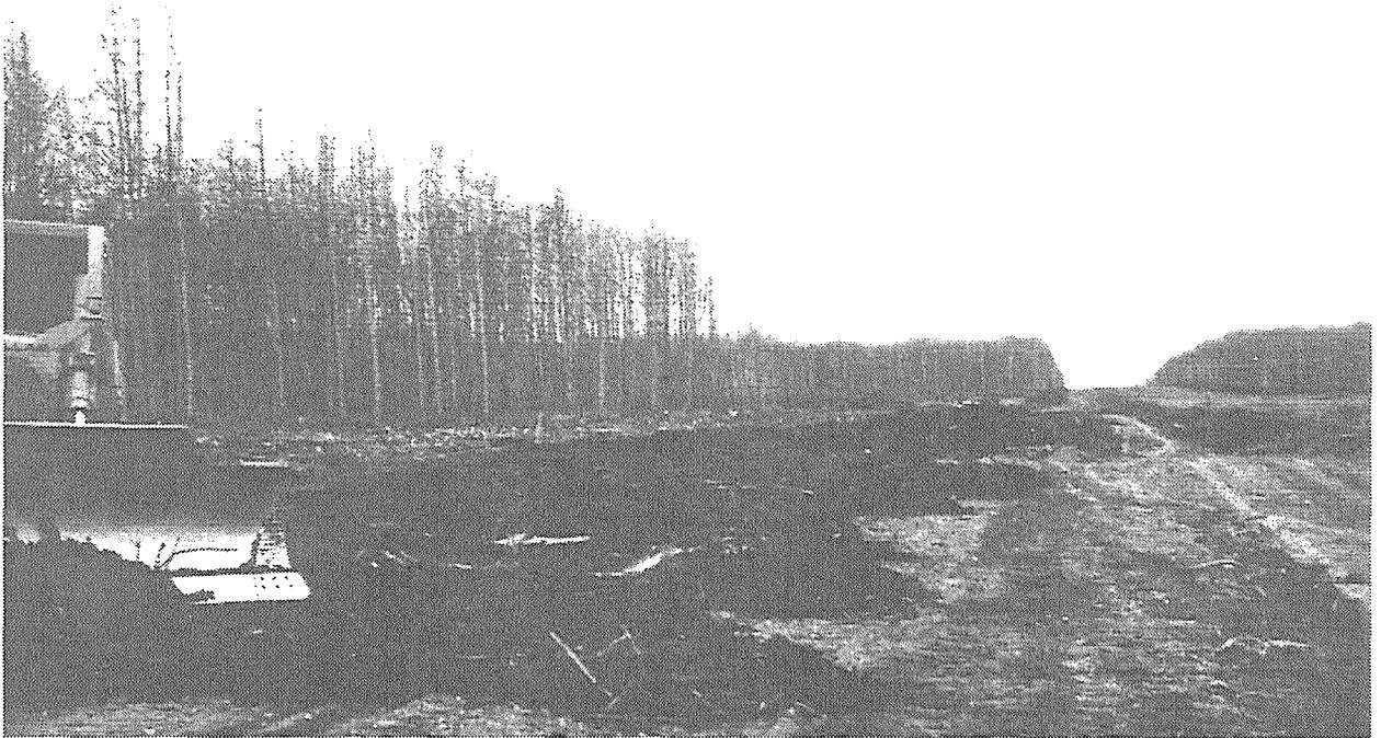
Photo 5. Topsoil replacement on 15 cm treatment.
