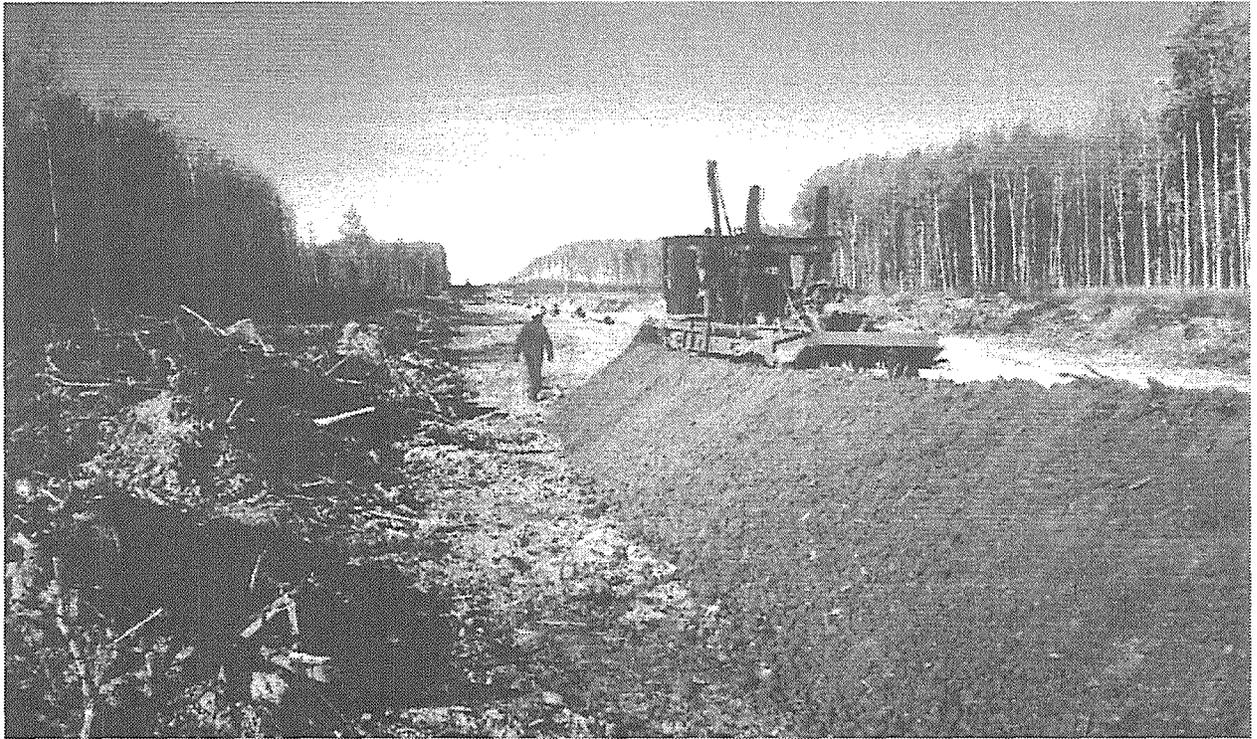
Photo 3. Wheel ditcher at work excavating trench.
