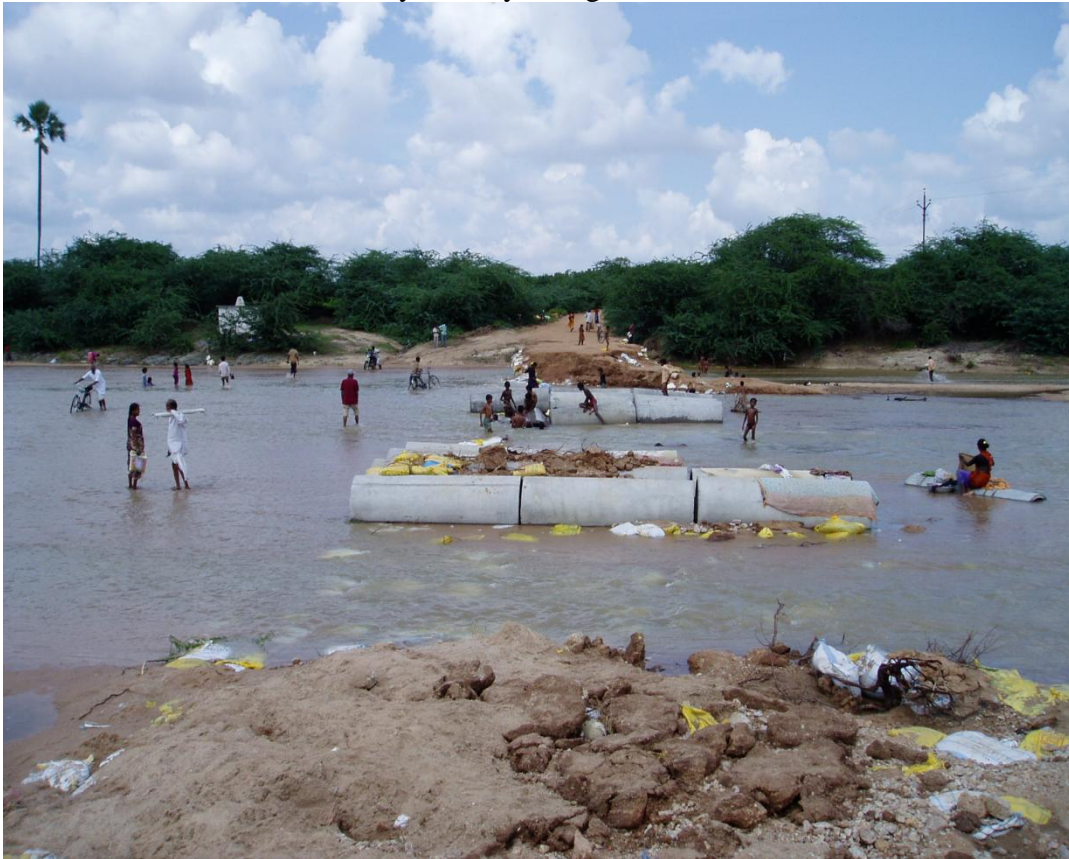
Picture 4.1: The washed away muddy bridge over the stream in Kadavendi.
