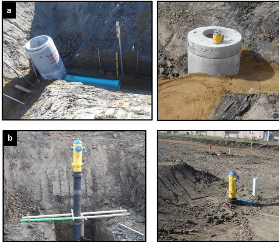
Figure 4-2-Main line installation by open cut: a) man hole & catch basin, b) fire hydrant
