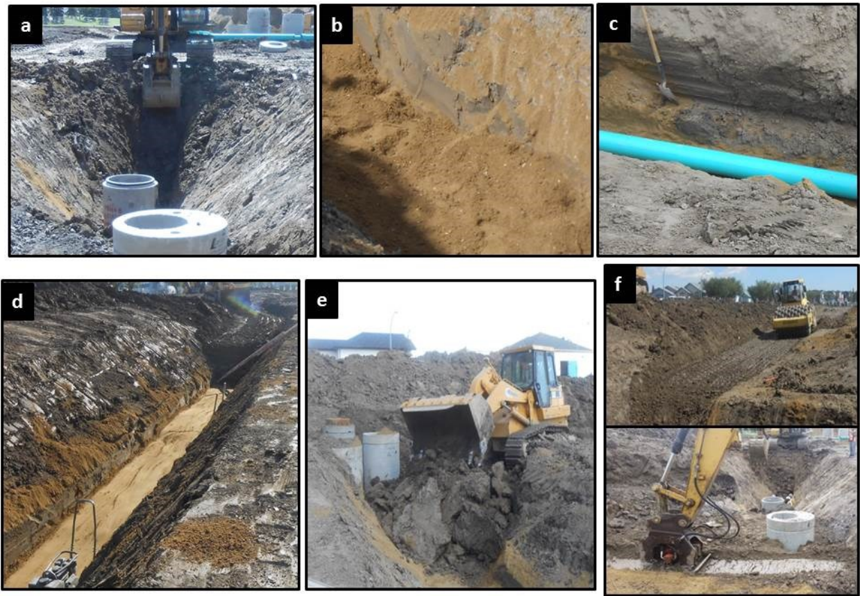
Figure 4-1-Main line installation by open cut: a) excavation, b) bedding, c) pipe installation, d) embedment, e) back fill, f) compaction
