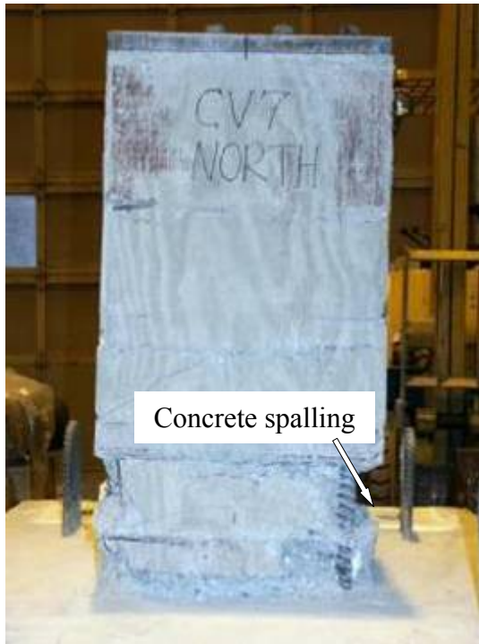
(e) At end of test (North side)
