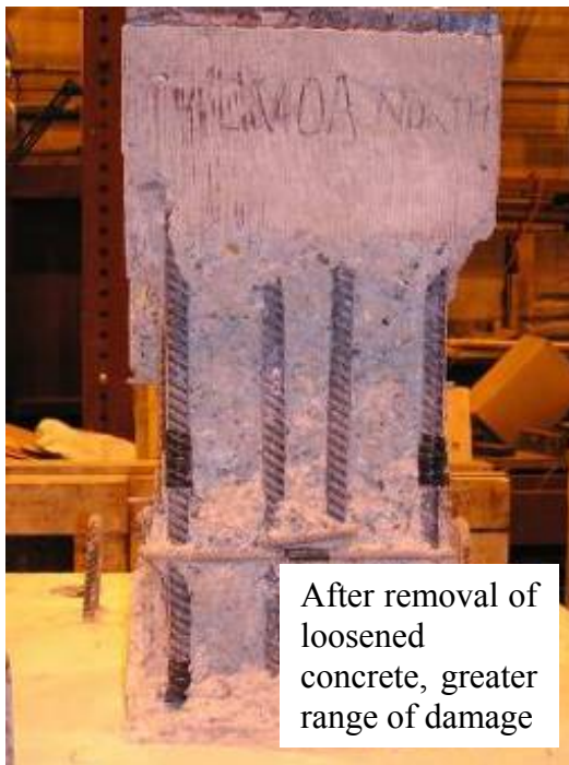
(c) At end of test (North side)
