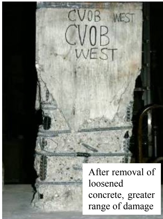
(e) At end of test (West side)
