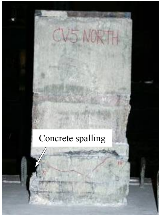
(e) At end of test (North side)
