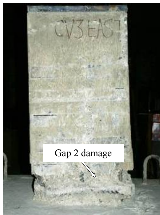
(h) At end of test (East side)
