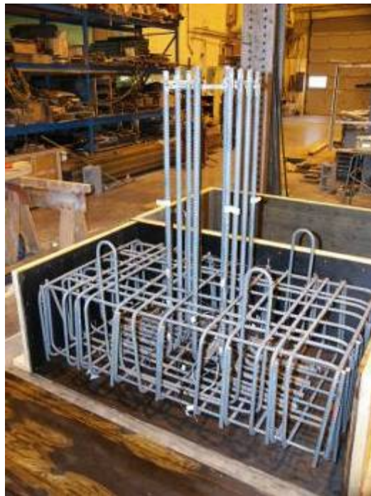
Figure 3-3 Rebar cage set in form
