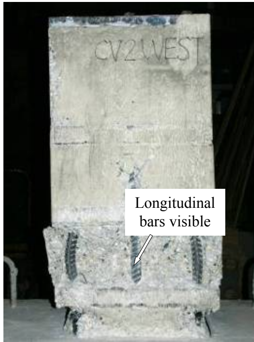
(e) At end of test (West side)
