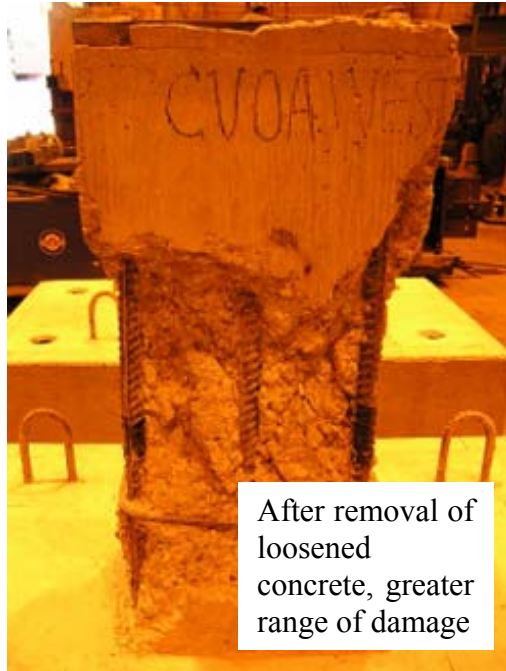
(e) At end of test (West side)
