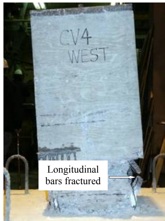
(e) At end of test (West side)
