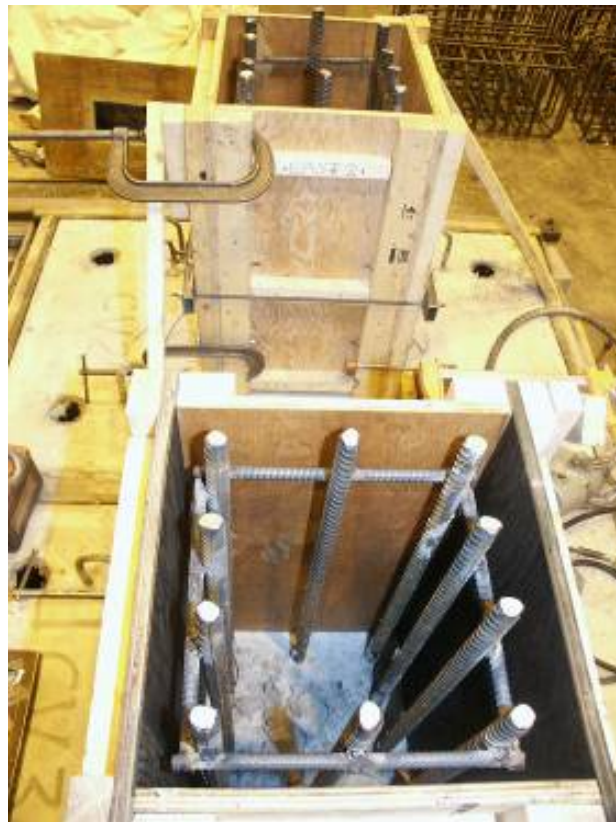
Figure 3-8 Two columns ready for concrete casting
