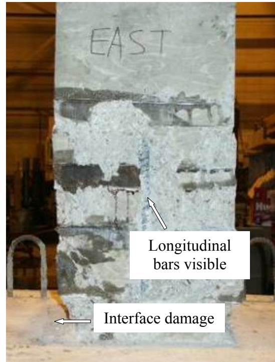
(h) At end of test (East side)
