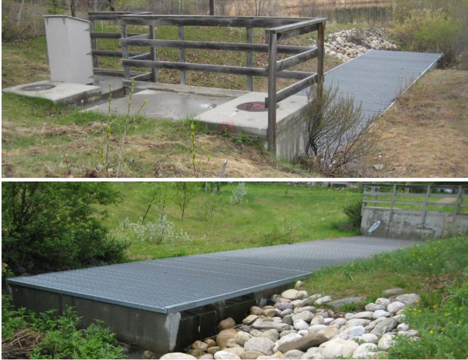
*Figure 3-3. The rectangular concrete sediment vault for first flush treatment in the inlet of the Rocky Ridge wetland.*
