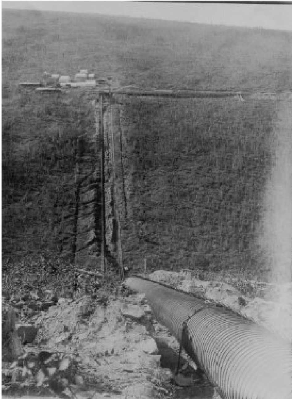
Image 5.14. Completed Yukon Ditch System, 1909. DCMA 1993.67.1.85
