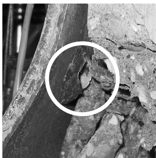
Figure 6-9 Weld Fractured from Link on the East Face (Column H3)
