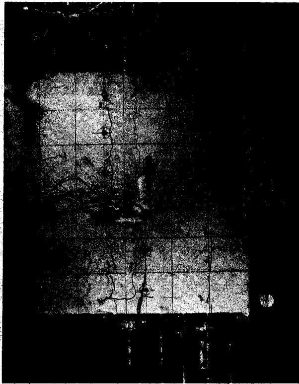
(c) Face A of Onset of Horizontal Cracking
