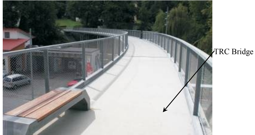
Figure 2.4- Pedestrian bridge made of textile reinforced concrete in Albstadt, Germany (Hegger et al., 2011)
