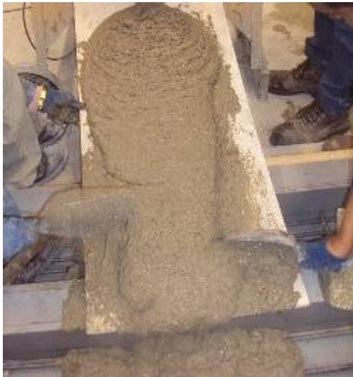
(a) Pouring and spreading of concrete
