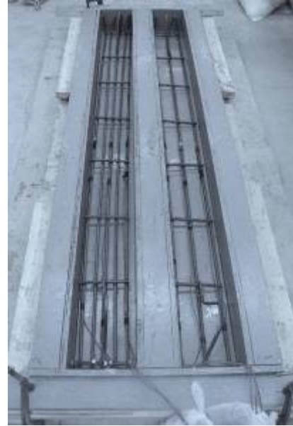
(b) Reinforcement cage
