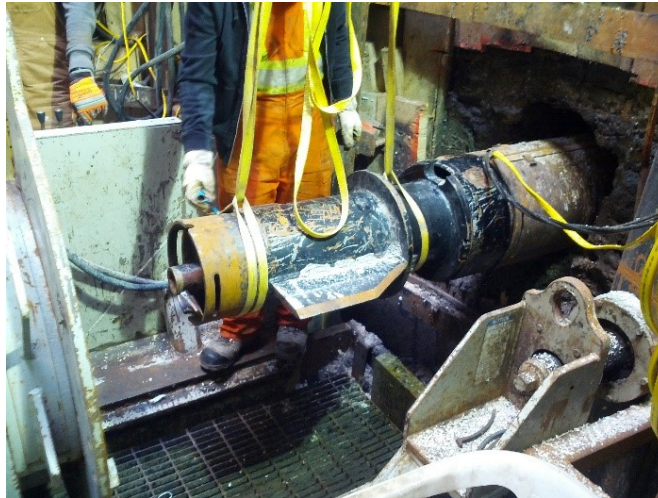
Figure 3.5. PCH adapter installation
