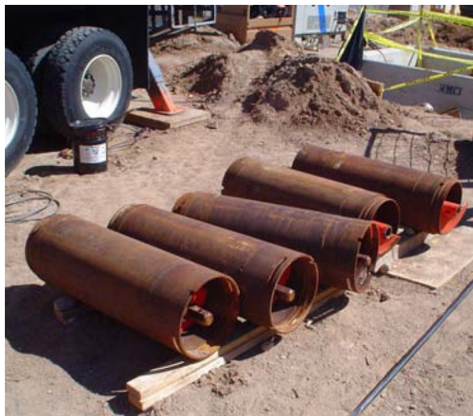
Figure 2.5. Auger casings placement on site (Boschert, 2007)
